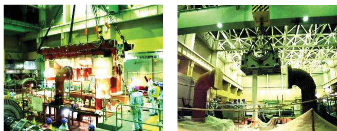
Fig. 5 Lifting of the HP casing and the bearing stand (Unit 2)
